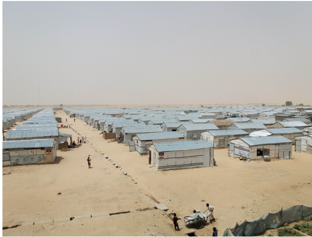
Figure 4.1: An example of an oblique angle image of Bakassi Camp, northeastern Nigeria Source: IOM
